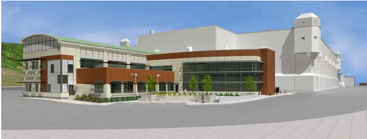
Fig. 5. The Uranium Processing Facility.
